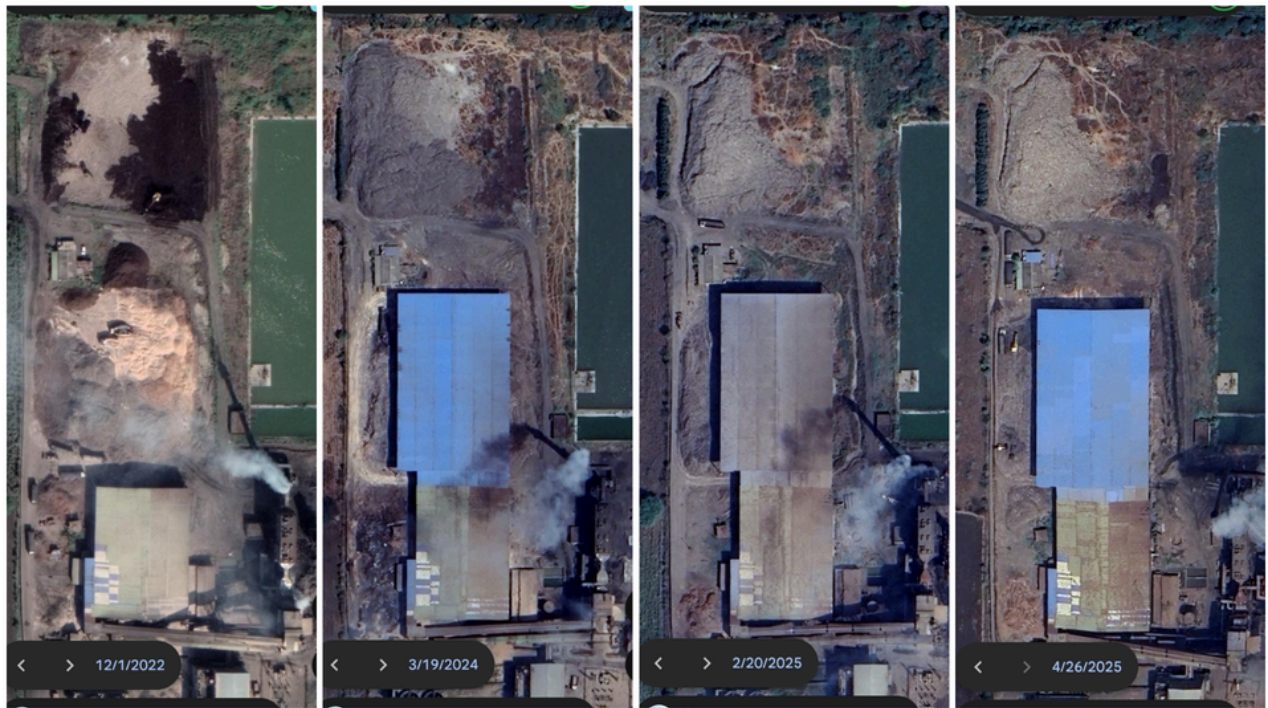
Figure 8- waste piling up (upper left corner)
